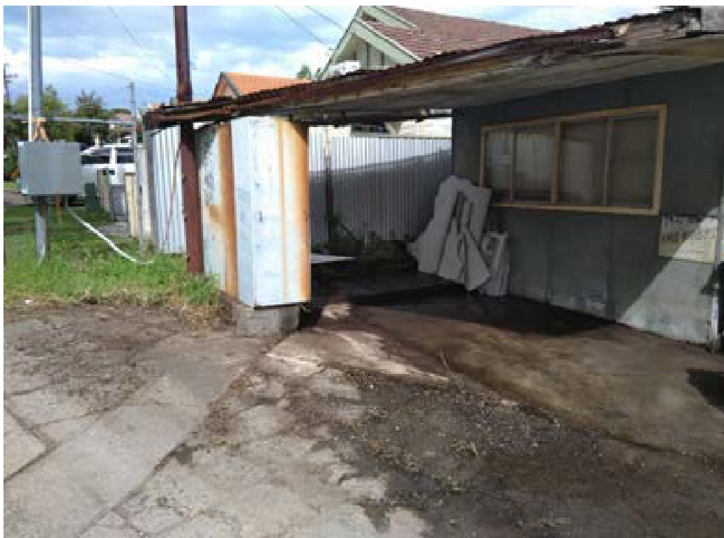
Photograph 3 - Site building with K-Weld sign visible, poor condition PACM and loose fibre cement sheets
