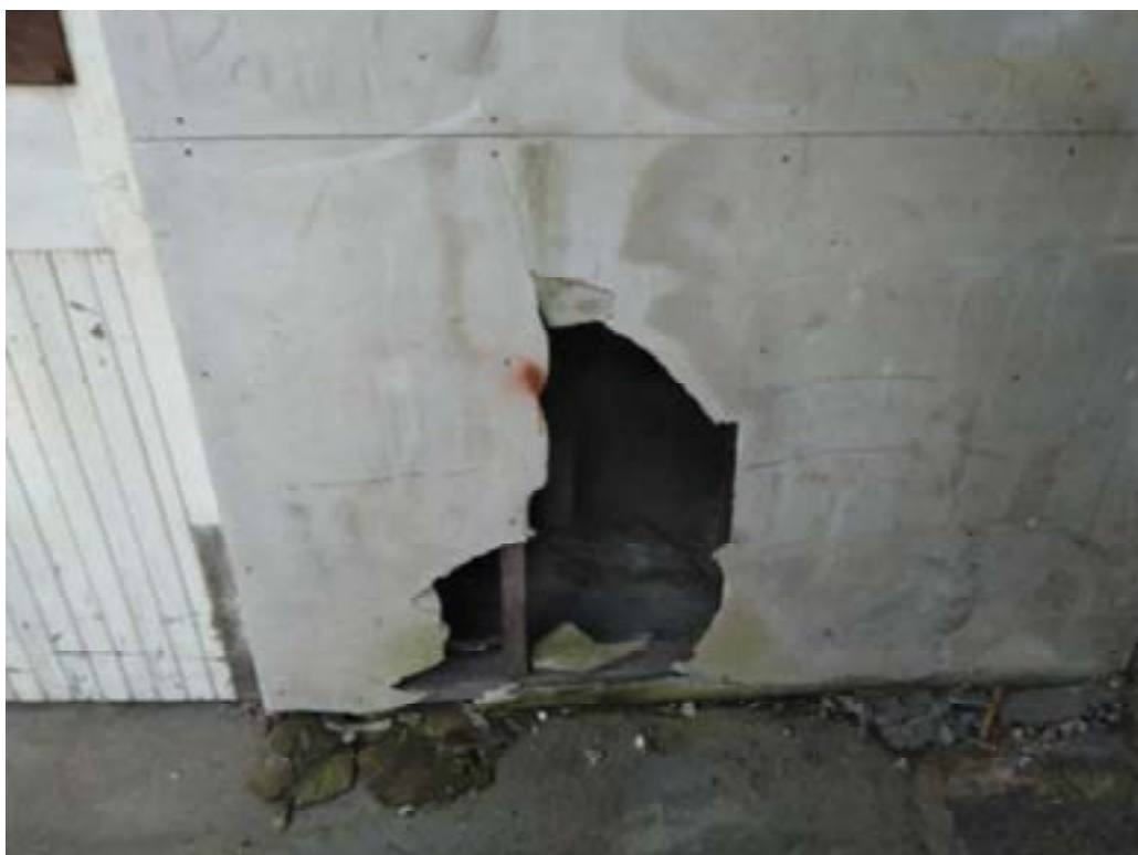
Photograph 5 - Damage to PACM wall of site building
