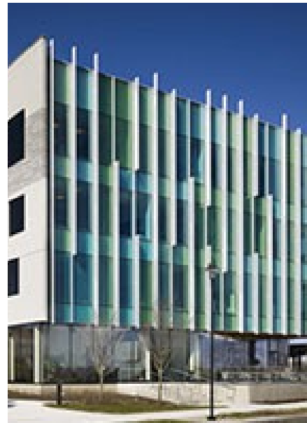
Vertical fins on glass facades
