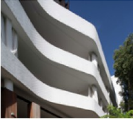
White rendered concrete balustrade
