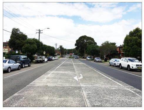
Brighton Avenue is a 30m wide street with a single travel + a parking lane in each direction. A bicycle lane is has been provided within the parking lane. The 30m width also accommodates a large median and wide footpaths on both sides of the street.
