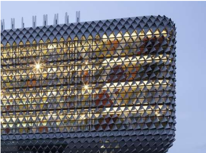
5/ SUNSHADING - OPTIMISED TO MINIMISE HEATLOAD + MAXIMISE NATURAL LIGHT
