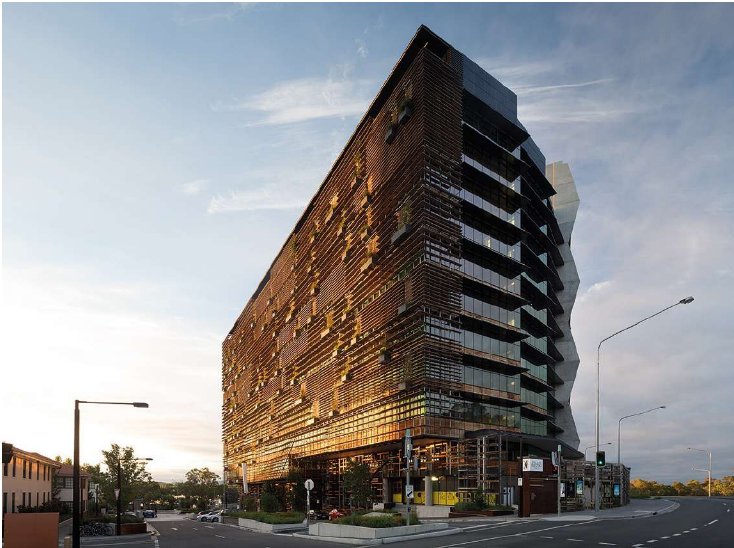
3/ FACADE SHADING - HEAT LOAD MANAGEMENT
