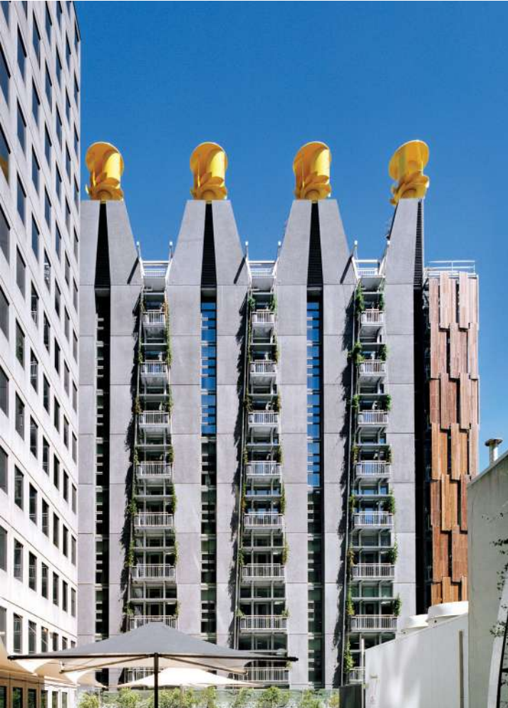
1/ WIND TURBINES - ENERGY GENERATION + ASSISTS NATURAL VENTILATION
