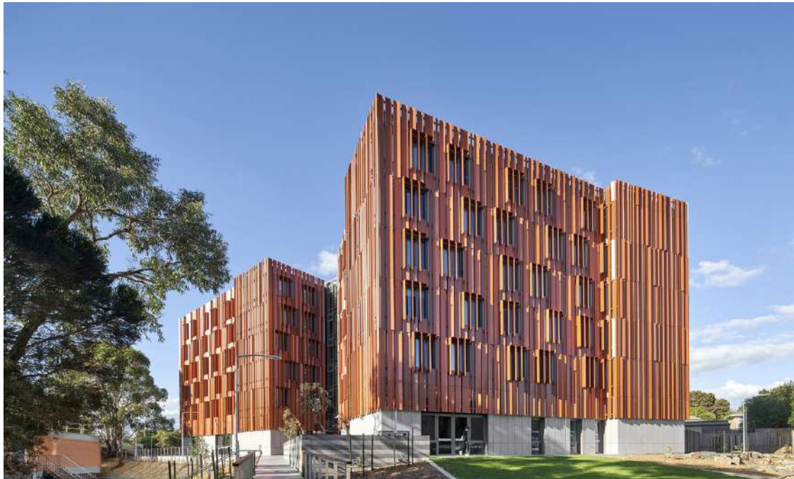
2/ 6 STOREY STUDENT HOUSING - PASSIVE HAUS + CLT TIMBER
