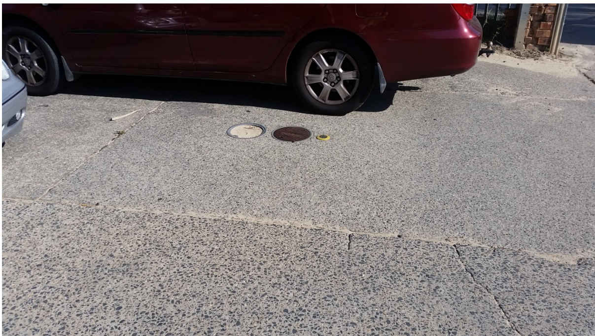
Photograph 8: Evidence of an underground diesel storage tank.
