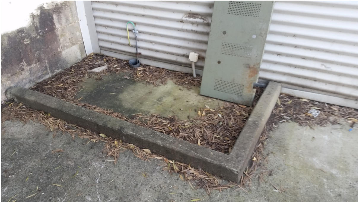
Photograph 5: Concrete bunded area with staining present at 23 – 25 Brighton Ave, Croydon Park.
