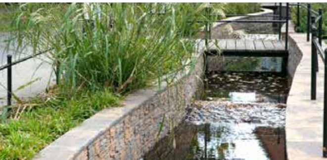
Introduction of rain gardens or swales next to a concrete encased stormwater channel
