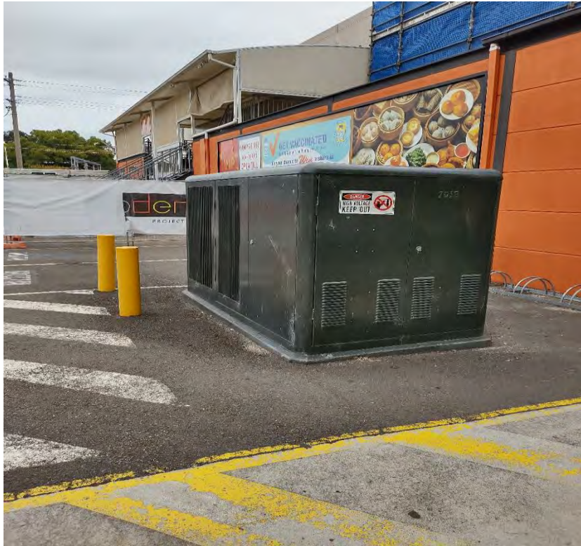
Photograph 1: Electrical transformer box
