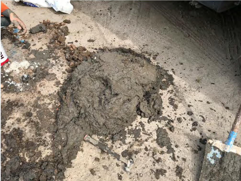
Photograph 9: Excess materials from MW06 borehole – former UST location. Borehole collapse on well installation due to instability.
