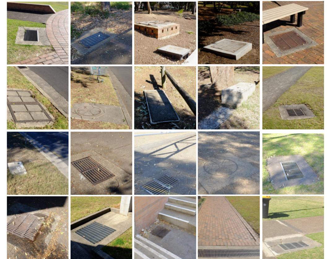
Stormwater pits are concentrated in the western portion of the park, in the amphitheatre and the carpark. Runoff from the eastern portions of the park, drains directly into the park ponds. Irrigation is limited to the amphitheatre lawn. There is no 3-phase power service in the park.
