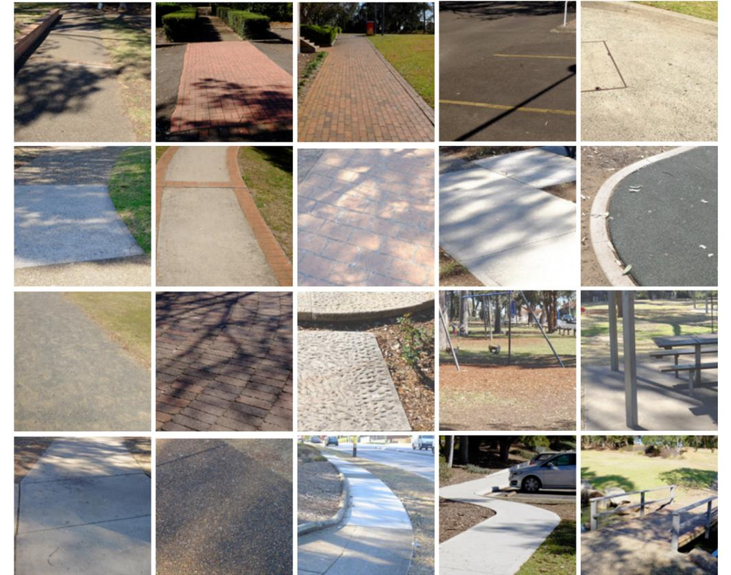
Park paths are combination of various materials and details, including pebblecrete, concrete, brick, asphalt and gravel. This paving is in varying condition and has been repaired poorly in various places. This wide range of finishes and inconsistent quality creates a disjointed and disconnected park character.
