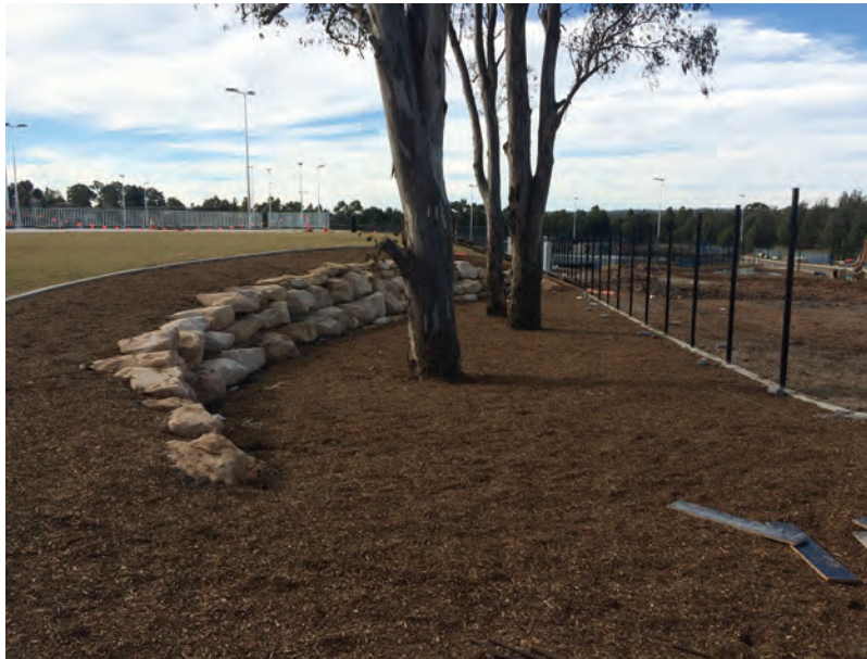
Example of rip rap walling enclosure for tree retention
